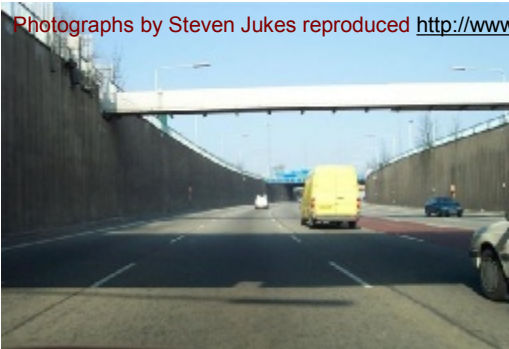
7 lane single carriageway
